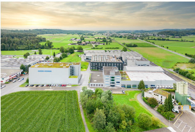
The new state-of-the-art production site in Pfäffikon ZH, Witzberg. Its rooftop is equipped with 866 photovoltaic modules producing 355,000 kWh annually.
